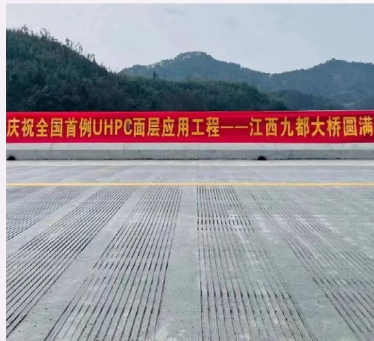
Chaokelong applied in the reconstruction of Jiudu Bridge in Shangrao's Dexing, Jiangxi Province
