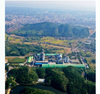
The "Beautiful Factory" construction of Xiangyang Factory
