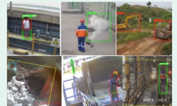
AI-based security monitoring system of Huaxin Cement
